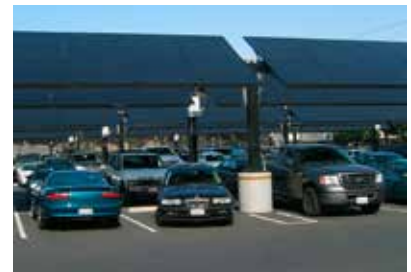
Solar panels utilized in parking lots can both generate electricity and provide shading for cars.
