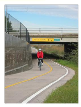
This cyclist has no margin of error on his right, and would benefit from an edge line on both sides. Although low, the bridge is higher than the minimal required vertical clearance of 8 feet.
