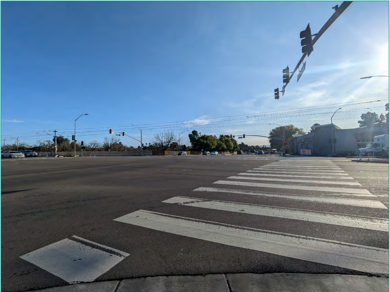
Figure 3. Long Crossing Distances at Hostetter Road and North Capitol Avenue Intersection
