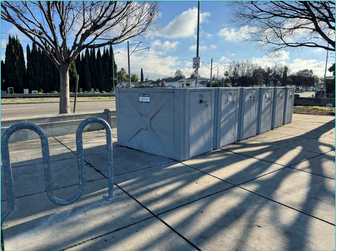
Figure 5. Hostetter Station Outdated Bike Lockers
