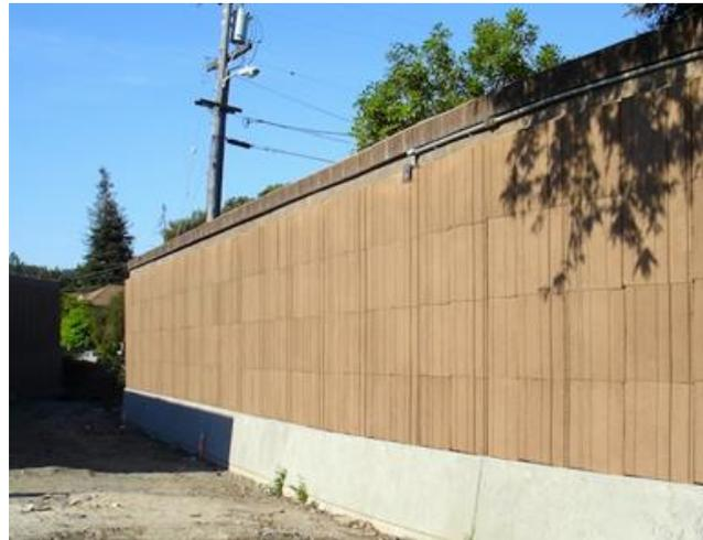
Figure 5-5: Acoustically Absorptive Barrier Tiles
