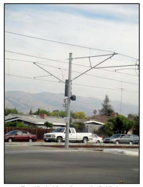
Figure 4 Overhead Contact System at Alum Rock Station
